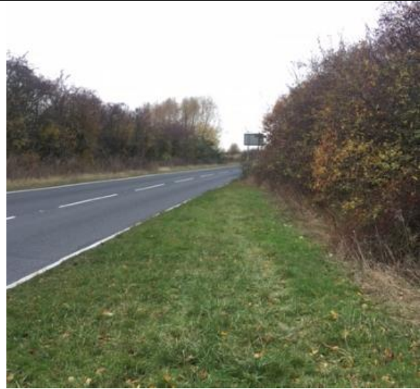
Image 2 – Old London Road; looking right out of junction in a northerly direction along Southend Road – restricted visibility
